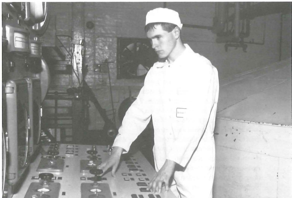
Mash temperature and time are constantly monitored from this mash-tun control panel.
